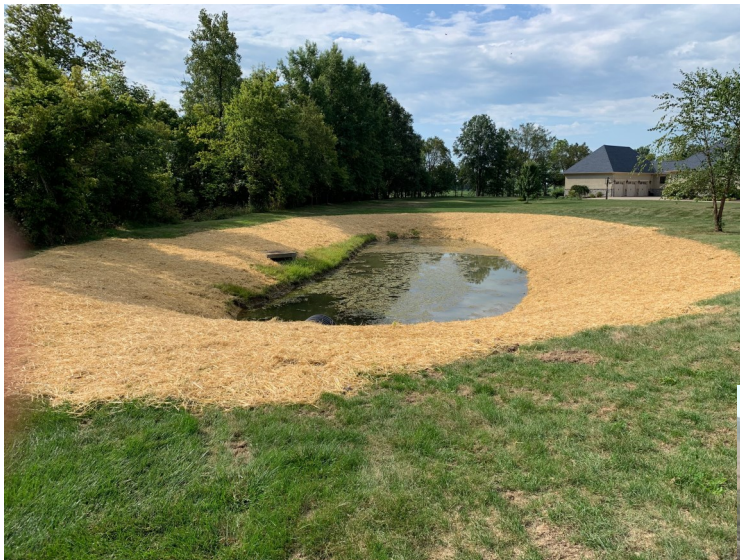
Picture show the finished product of a basin clean out in Autumn Ridge Subdivision. Scheduled sediment removal along with damage by muskrats were causing drainage issues in the area.
