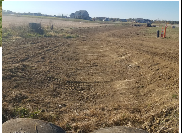
Picture shows the final surface grade work after a tile main replacement in the Pleasantview Farms Subdivision. This work was completed in cooperation with Darby Twp. trustees.
